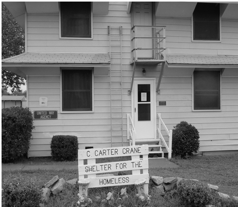
A two-story wooden barracks that once served as home for soldiers training at Ft. Sill now provides a safe and clean temporary residence for homeless people in Lawton. Great Plains Improvement Foundation operates the 4,000 square foot C. Carter Crane Shelter for the Homeless.
