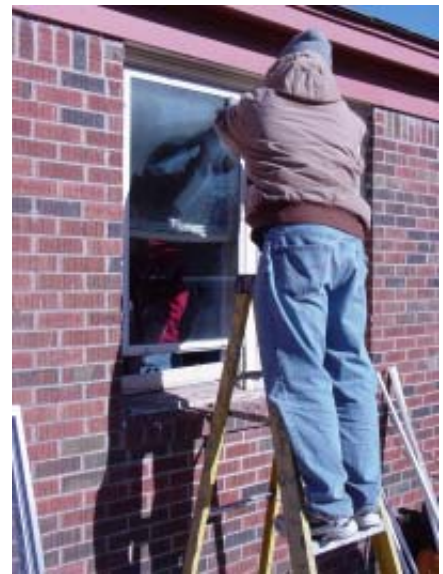
Window replacement is sometimes required to stop air infiltration into a home.
