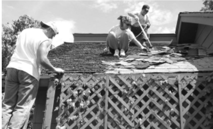
Campers replaced roofs on five houses during the week-long WorkCamp.
