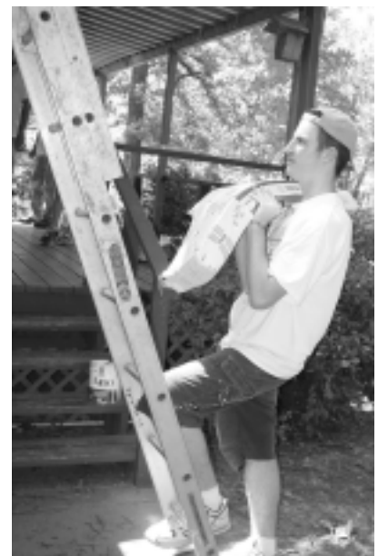
This camper lugs shingles up a ladder in Jay.
