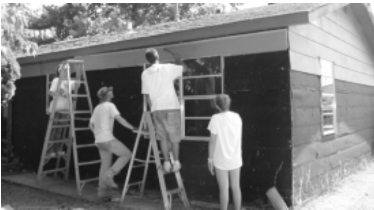
Campers replaced siding at several of the houses during the Workcamp.
