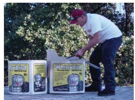
Trayler Pitts installs ventilators in the roof.
