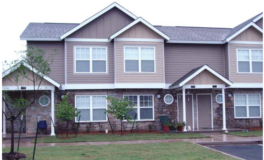
One year after breaking ground for construction of a multifamily housing complex in Pawnee, the project has been completed and is filled with tenants. United Community Action Program was the developer for the project.
